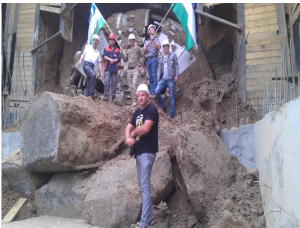
Fig. 5: Successful exit of the TBM into the dismantling chamber. When the tunneling is completed, surveyors and builders
