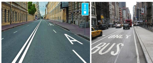
Fig. 4: Arrangement lane reserved for public transport
