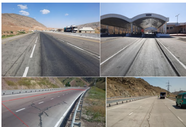
Fig. 2: The results of the negative impact of the movement of trucks with overload on the roads of the Republic of Uzbekistan
